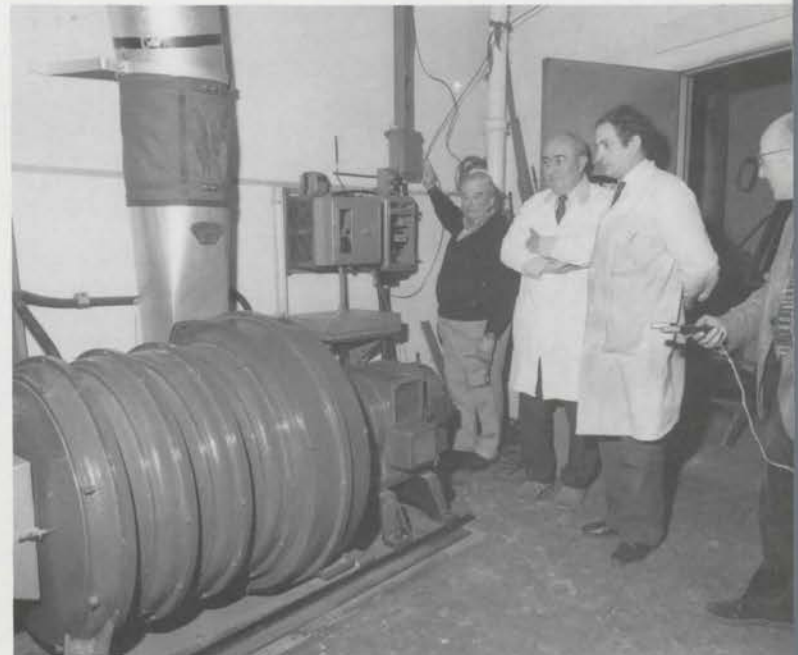
The blower, a British-made "Discus" unit, is switched on for the first time, an event which was recorded.
