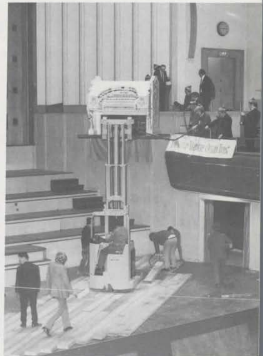
Almost there! Lifting the console to its position at circle level in the Free Trade Hall.
