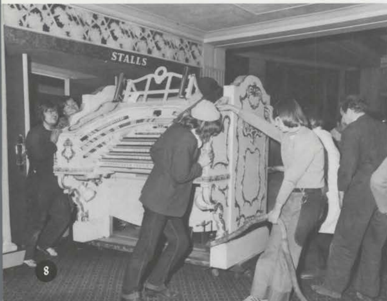
The console emerges into the lobby.
