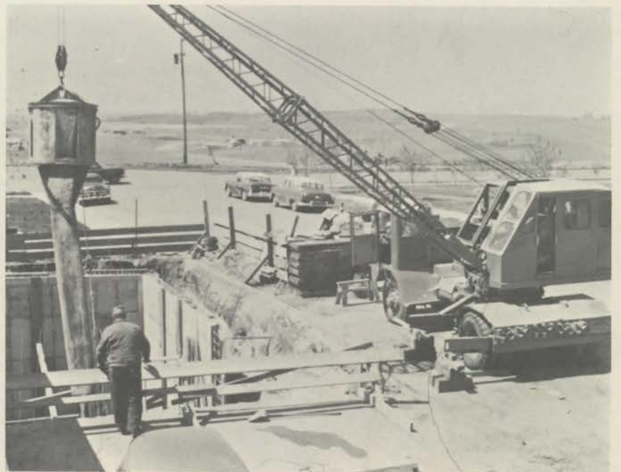
Solo walls are poured, footings for main chambers are being poured.
