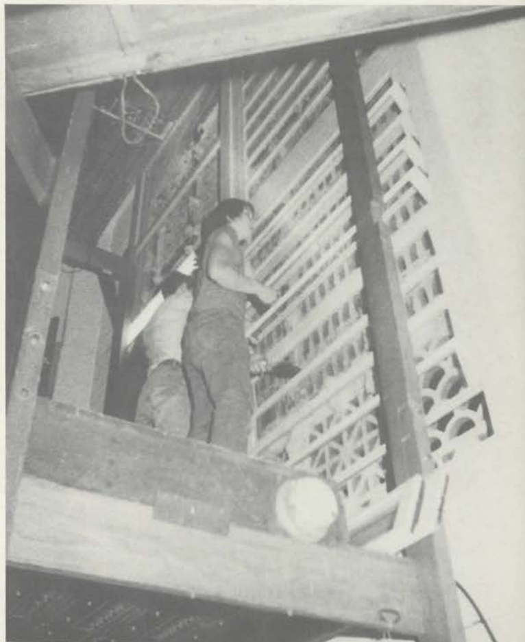
David Junchen and Dan Homberger work on glass swell shades prior to racking pipe-work in Solo chamber.
