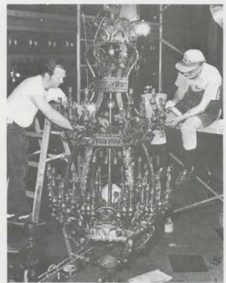
Richard Parker and Bob Johnson complete re-wiring of the main chandelier in the grand lobby of The Alabama Theatre. Each broken piece of glass was exactly duplicated and every wire was replaced.
