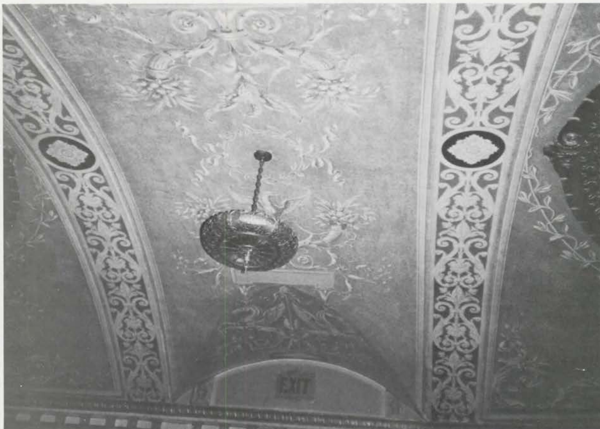
Ceiling decorations beneath balcony are all 100% restored.
