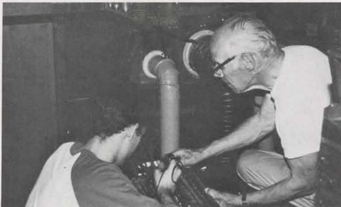
Soldering connections being separated here by Doug Barnhart and Lawrence Frazer.
