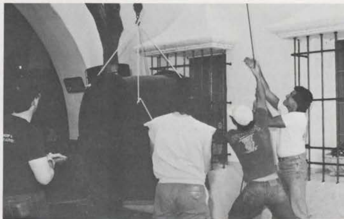
Hoisting the giant blower into the Arlington.
