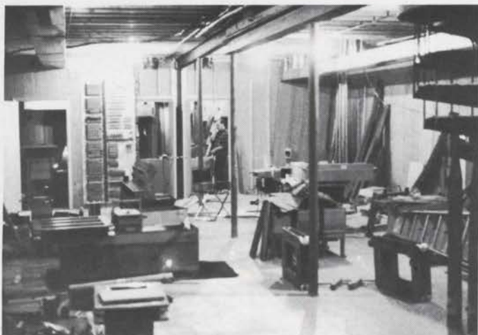
Work well underway, Dan Stankey stands in one chamber.
