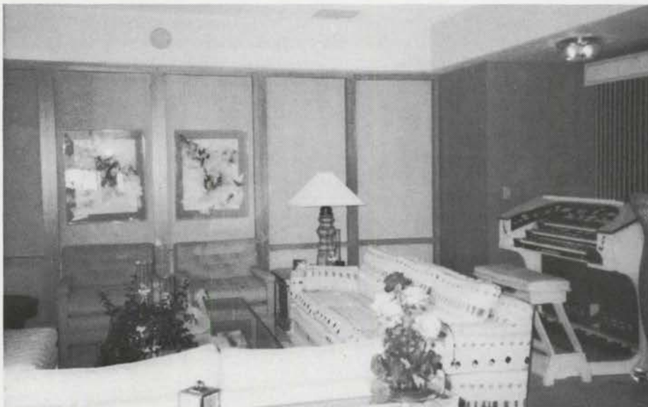
Paneled wall conceals organ chamber. Entry is gained through panel nearest the console. The wall forming the left side of the console alcove is part of the chamber and contains relay components. The chamber measures four feet deep, eight feet high and approximately 25 feet long.
