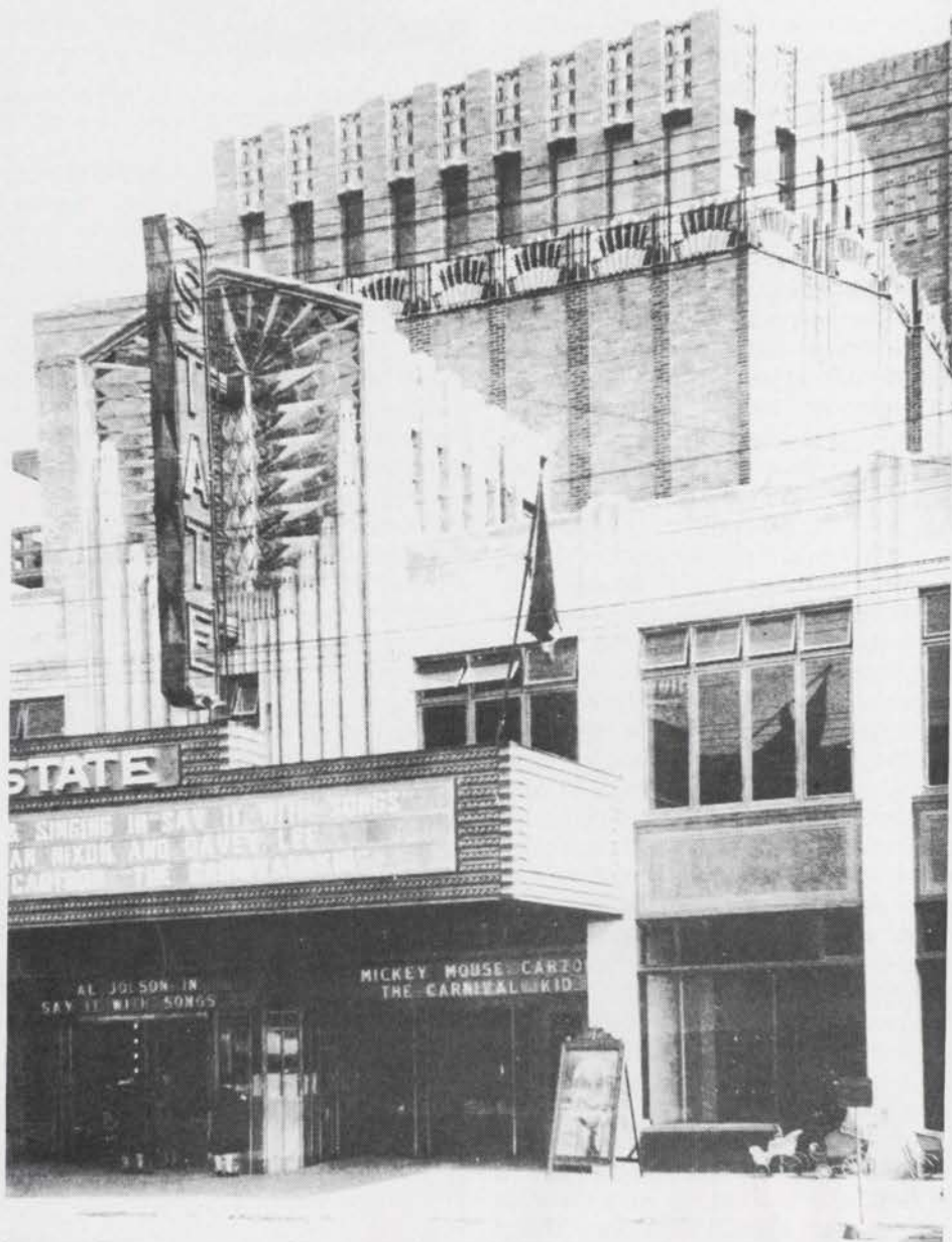
Original exterior of the State Theatre. Each decorative raised surface behind the vertical sign and within the four "wedding-cake" levels was silhouette illuminated at night. Glazer photo
