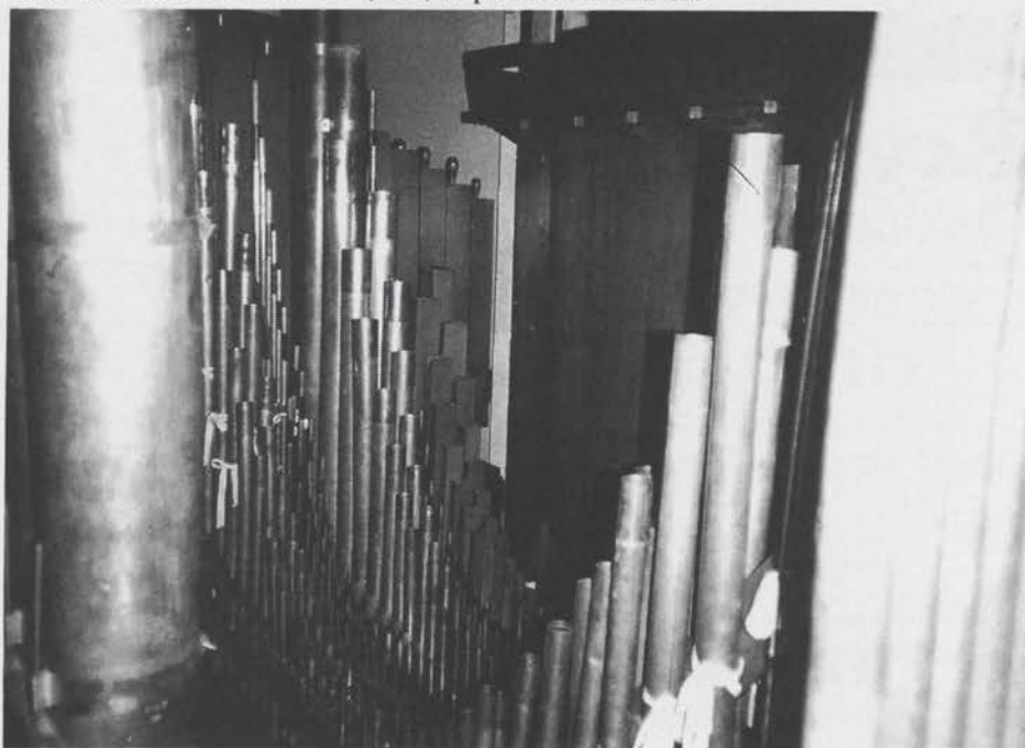
Main Chamber in FOX-Hanford 16' (metal) Diaphone is to extreme left.
