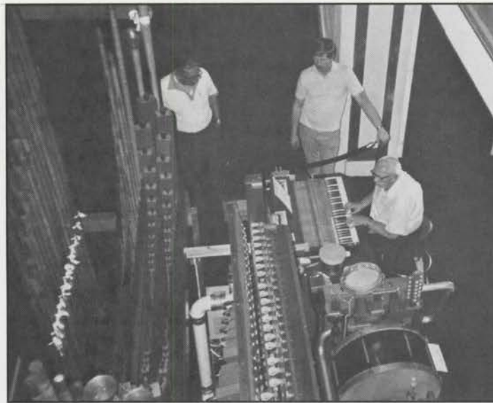
LOBBY DISPLAY ORGAN —Viewed from the mezzanine level of the Chambersburg, Pa. Capitol Theatre, Max Cooley, right, plays on keyboard wired to Flute and String ranks of pipes, harp and toy counter, which is one-seventh of the Capitol's Moller organ now under restoration. Restoration crew members Gil Singer and Mark Cooley look on.
