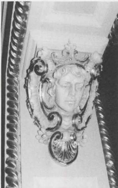
Restored decorative plaster.
