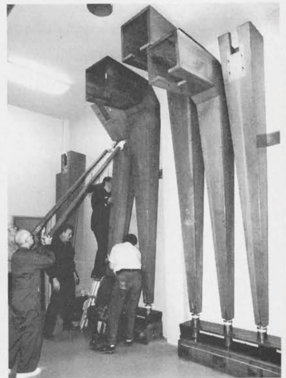
Erecting the 16' Bombarde in the Perfound chamber. The tallest pipe cleared the ceiling by 1/2". It was not necessary to do any additional metering of any pipes in the organ.
