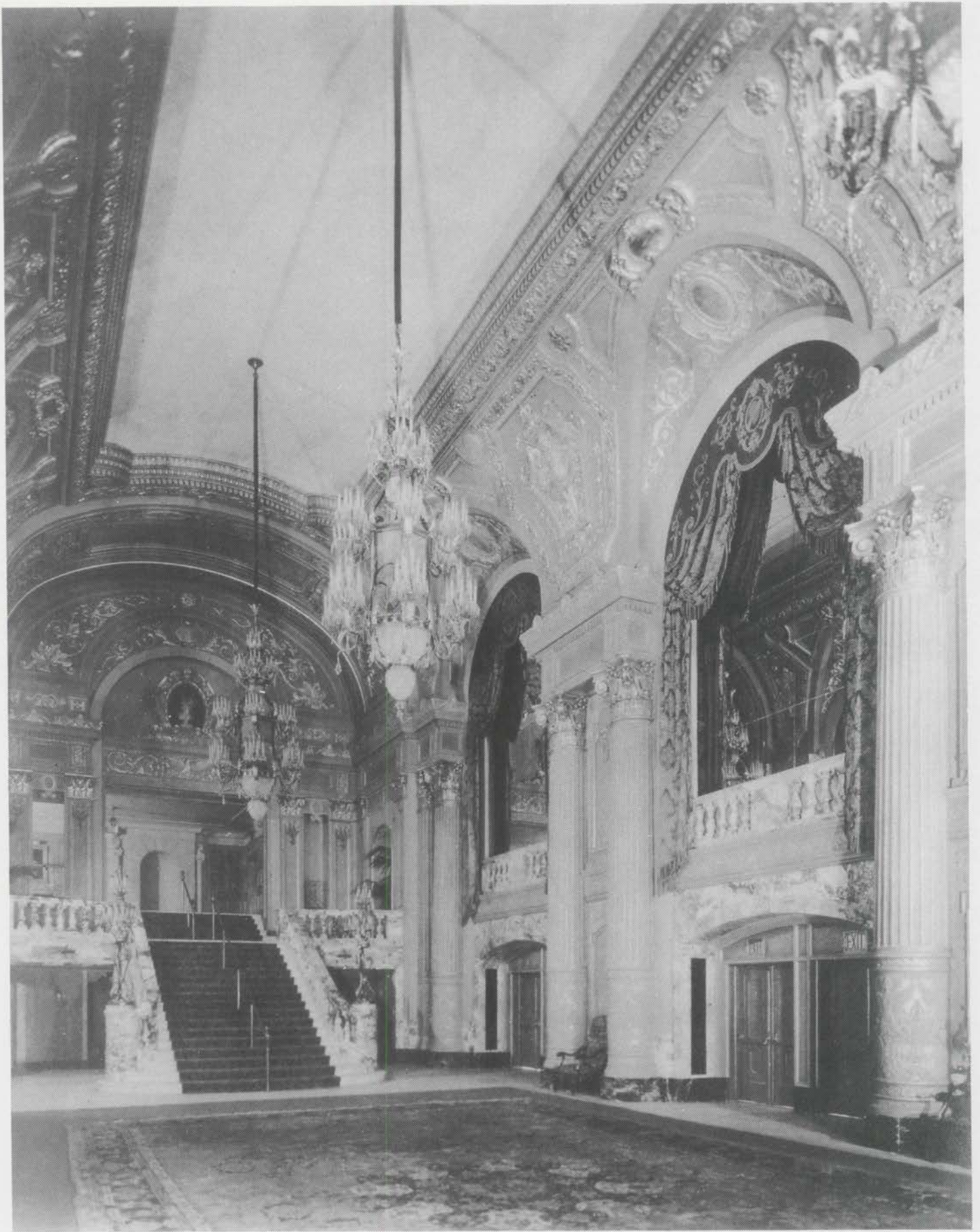
The innermost and largest lobby is here shown before the ceiling mural was installed. Behind the staircase was a bank of elevators.
