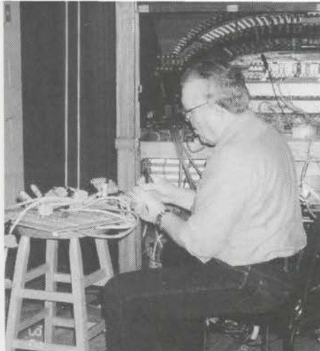
Herman Thompson concentrates on wiring a junction board.
