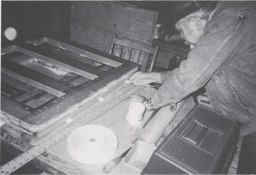
Ray Anderson putting new hinges on regulators.
