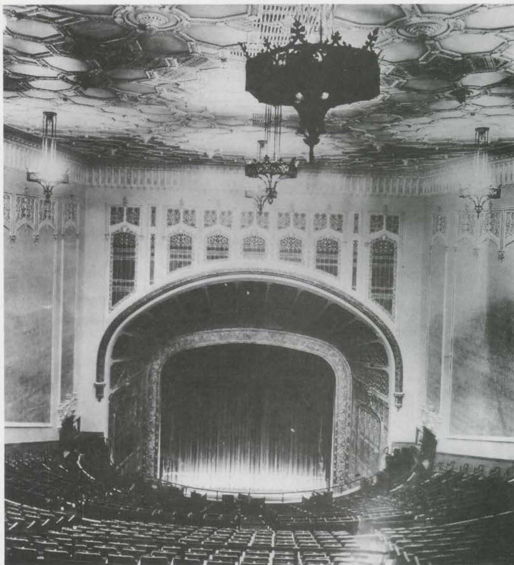
The entire disposition of the organ is visible here: Main and Solo in their usual places, Foundation and Tuba above the proscenium, Echo well back in the ceiling. The piano and xylophone stood atop the Main, the 32' Diaphones over the Solo. E.M Stout Collection
