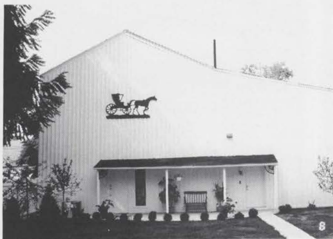
Exterior of the Carriage House.
