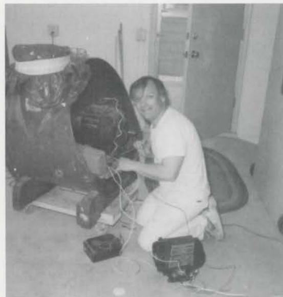
Bob Markworth investigates a balky blower motor. Tom Jeffery photo
