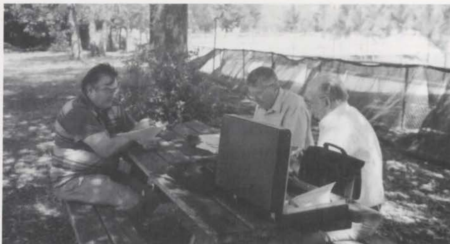
Ted Campbell (left), Ed Nielsen (right rear), and Red Carlson of Artisan Instruments, go over the final phase of the electronic relay installation.
