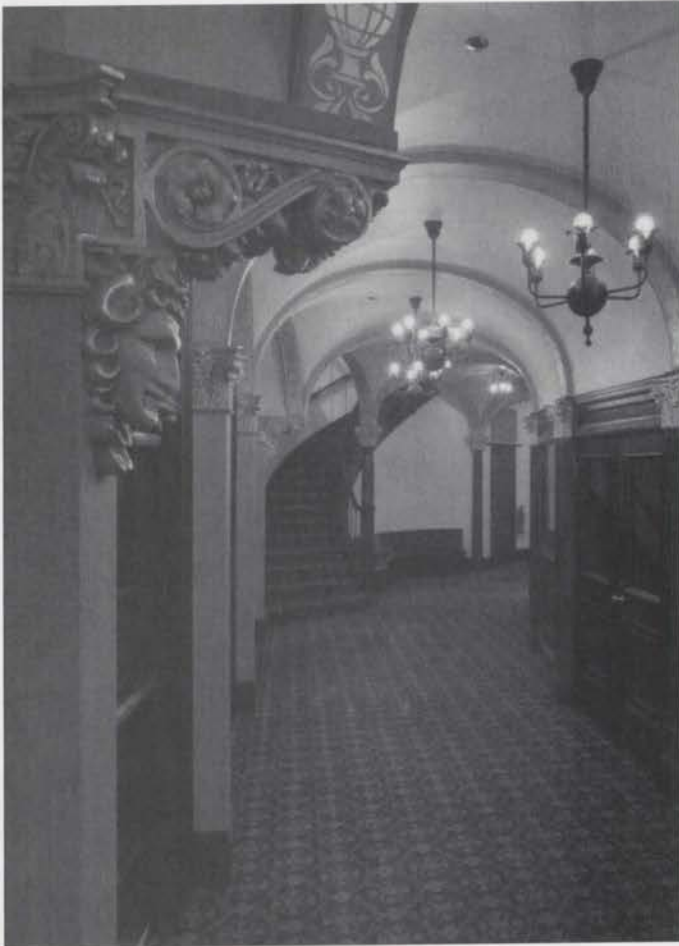
Inner foyer with curved staircase, gilded plasterwork, and mahogany paneling. ©1989 Phil Revoir. Used with permission.
