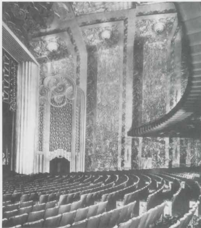
The sidewalls, less complex than they appear, are assembled from only five original models, plus trim pieces, arranged differently on each vertical section. All of them appear in the panel between the organ grille and balcony rail. Steve Levin Collection
