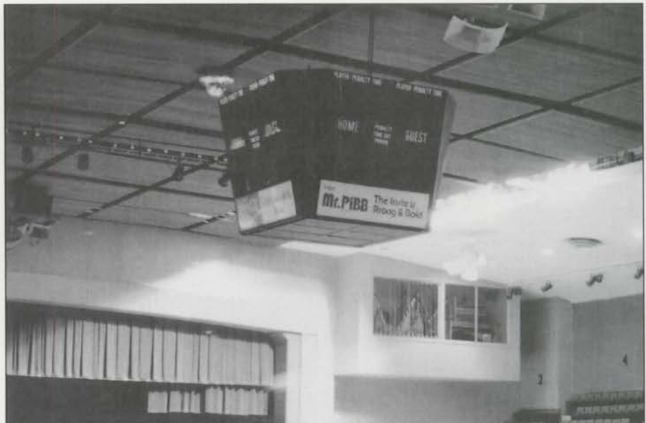
Sioux City's municipal auditorium. One pipe chamber is to the right of the proscenium, and the console platform is over an entrance tunnel. Tom Jeffery photo
