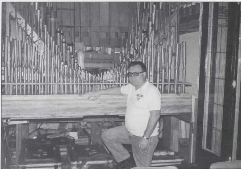
Larry Ferguson in Kimball pipe chamber. Bill Daniels photo
