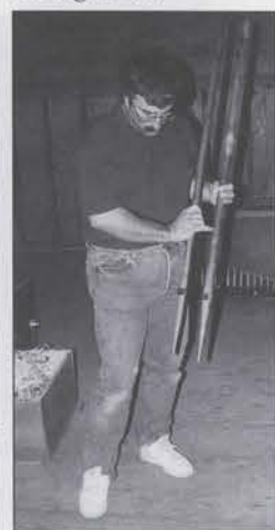
Center: Tom DeLay comparing pipe scales of two Morton Violins; left 1921, right 1927 larger scale. Both 10' wind pressure.
