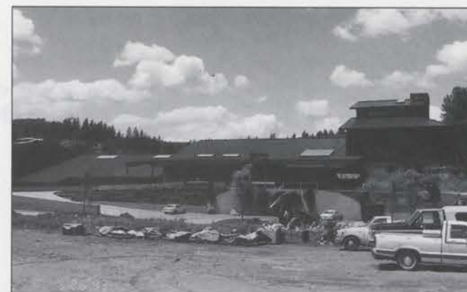
Looking north at the overall winery complex. The organ listening area is the central complex
