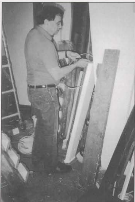
Warren Thomas working on lighting system for Main chamber.
