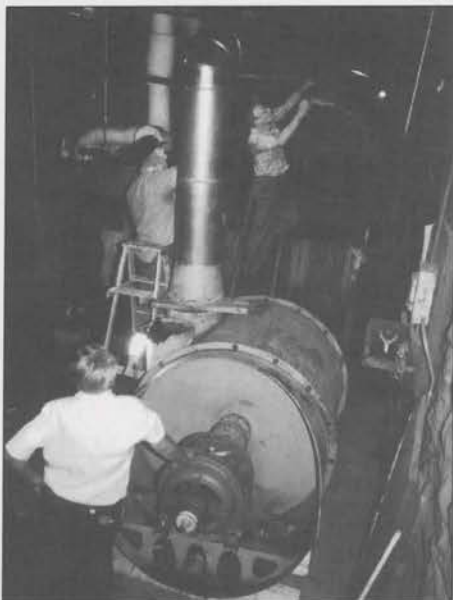
20 H.P. Orgoblo installed with windline being connected.
