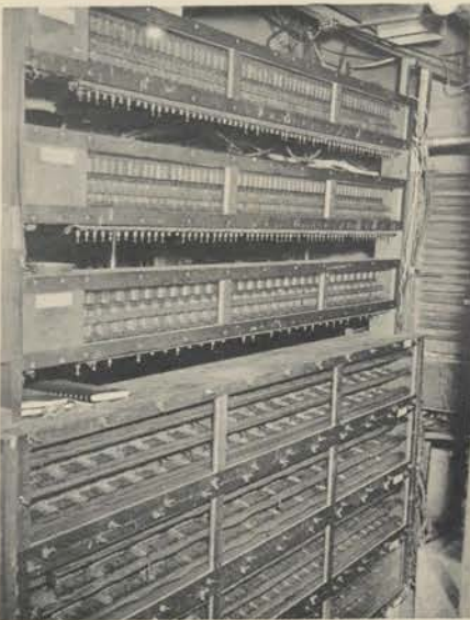
Photo shows Relay Room in Harold Logan Wurlitzer installation.
