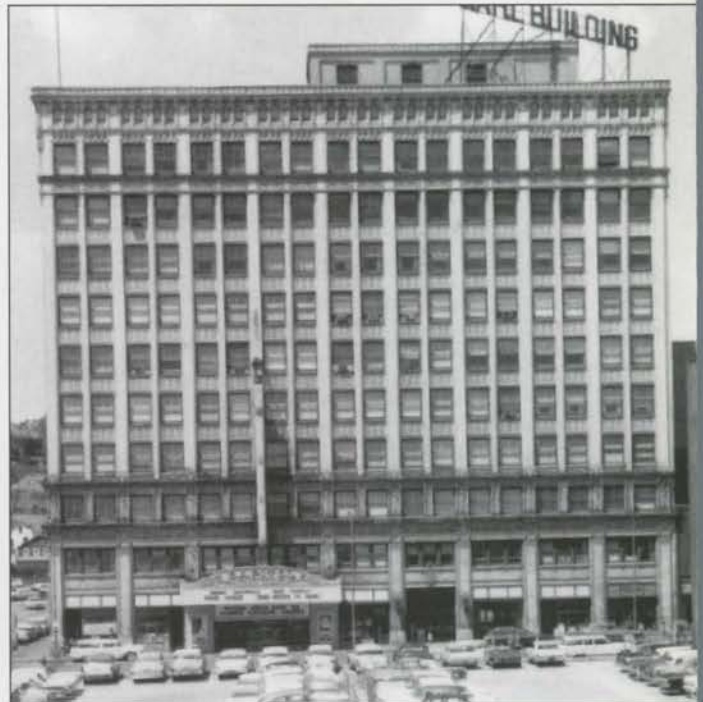
The Kahl Building, home of Davenport's Capitol Theatre and its Wicks Pipe Organ, was a Christmas gift to a local college.
