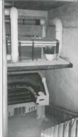
Concrete stairwell utilized for reservoirs and storage of Kimball console. Jinny Vanore photo
