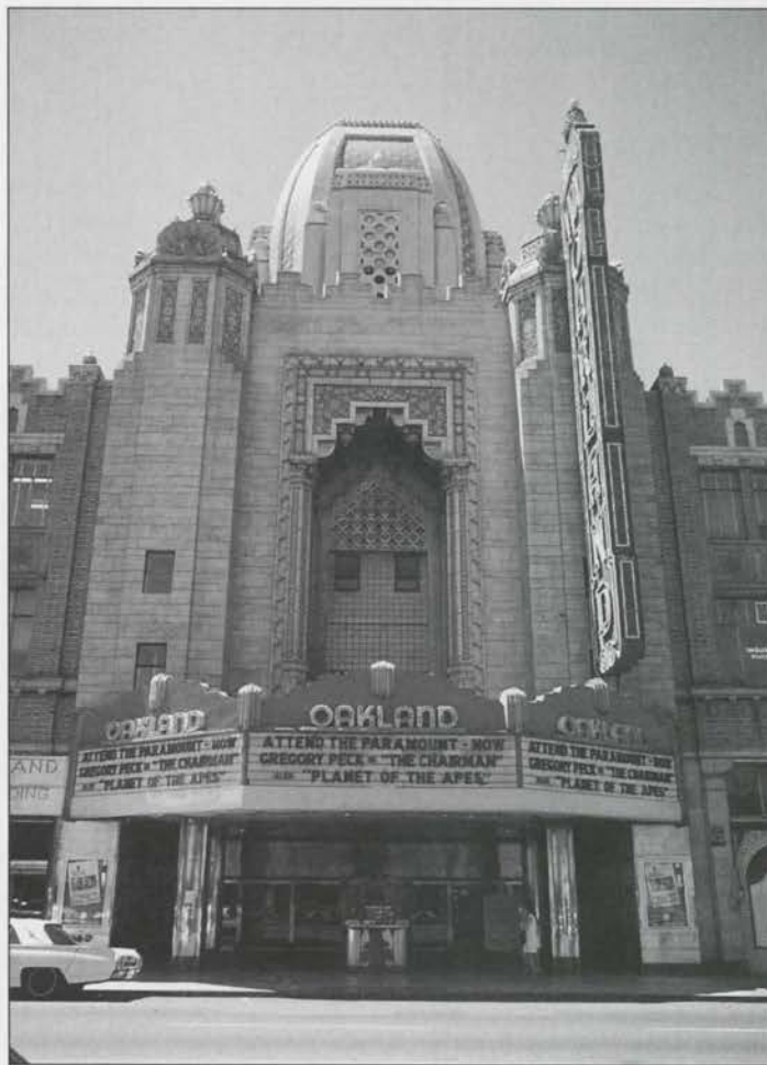
The facade in its present form, with what's left of the 40s neon marquee. The glass bricks above the sign replaced a stained glass window in the Moorish manner. Steve Levin Collection
