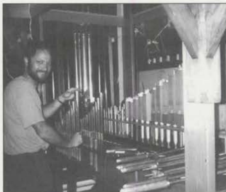
Organ Crew Chief Greg Breed installing last of pipework in chamber.
