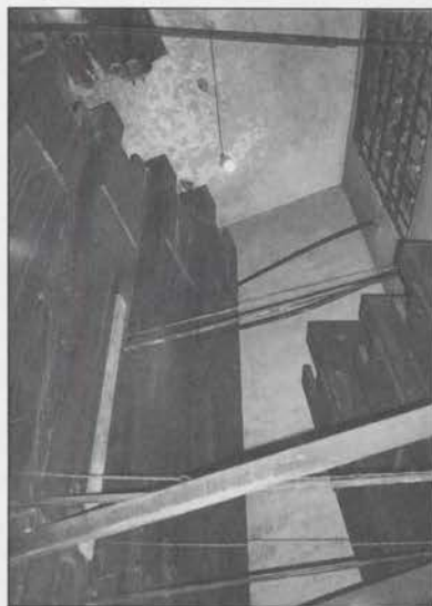
View up to the tops of the 32' Diaphones. Notice the small grille to the left.
