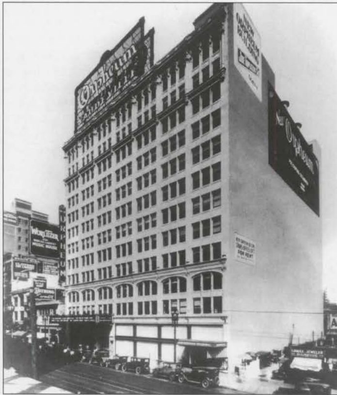
Lansburgh's usually unerring eye for scale and proportion deserted him on the marquee: it's too small and set too high. The present neon trapezoid is far more effective. Note the Wurlitzer Building up the street.
