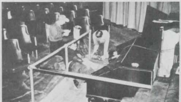
Kagy, Meier and Arey hard at it replacing flooring and installing protective rail around the console.
