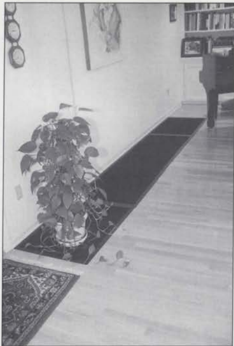
Tone chute grille opening into the music room. Below: Chrysoglott and chimes installed on balcony.
