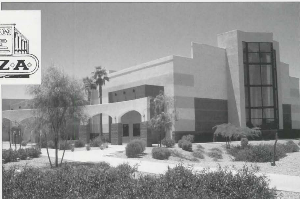
The Organ Stop facility has a very contemporary look. The organ blowers and diaphones are visually displayed for public appeal.
