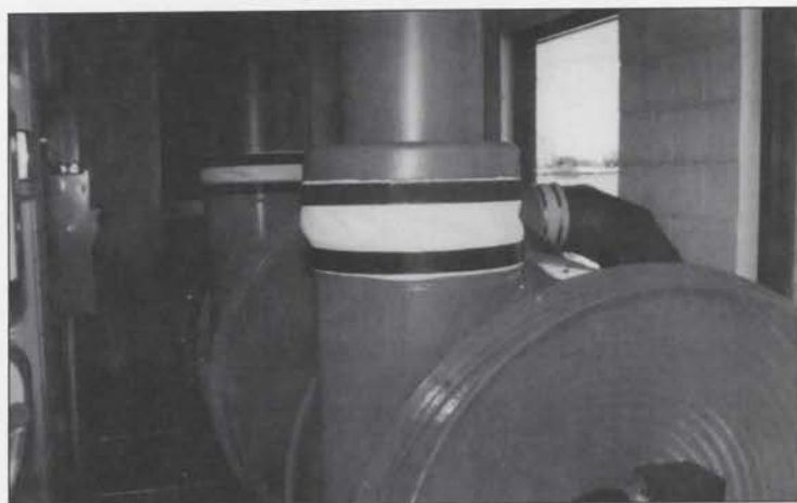
All lined up in a row ... The four Spencer turbines are capable of producing over 11,500 CFM of static wind.
