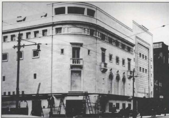
The Granada/Gaumont, Manchester under construction in 1935. John B. Potter photo
