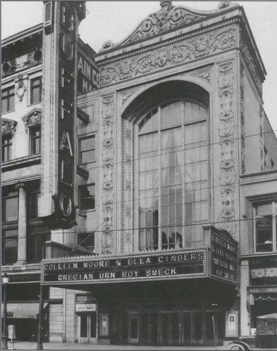
Tall windows were almost always part of a Rapp facade. The composition was stronger before most of the terra-cotta above the window was removed. Note how the vertical draws attention away from the asymmetrical arrangement.
