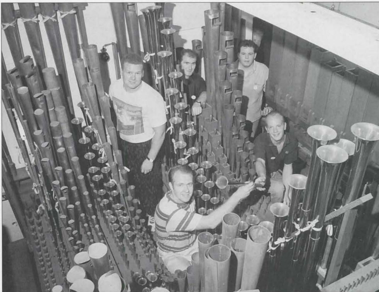
August 19, 1997 ... the first pipe is removed from the Solo Chamber.
