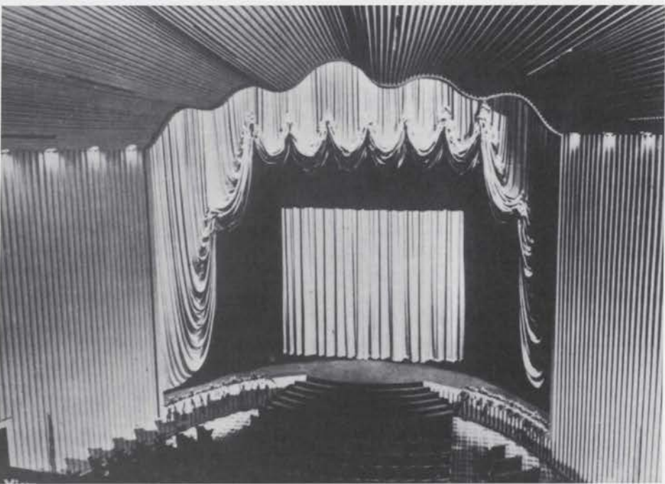
The 1942 transformation of the El Capitan Theatre in Hollywood from a legitimate stage theatre to a movie theatre, and renamed the Paramount, included a complete renovation, including a modern streamlined facade (top) and an interior cloak concealing the ornately decorated auditorium (above) originally designed by renowned theatre architect G. Albert Lansburgh.
