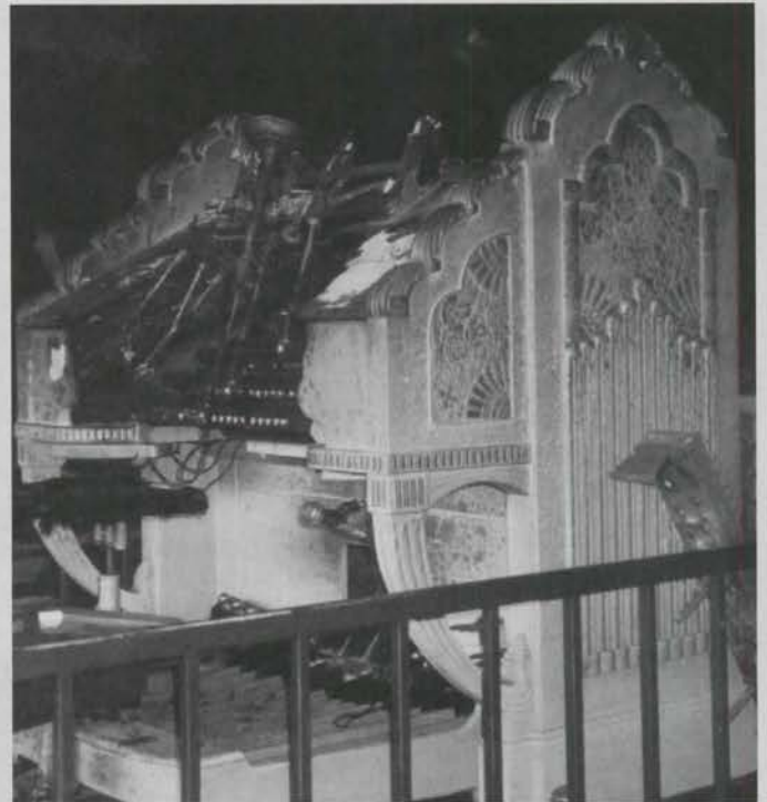
The burned console. The shell remained essentially intact, but the stoptabs, keys and interior workings melted from the heat. Damage occurred from heat, smoke and water.
