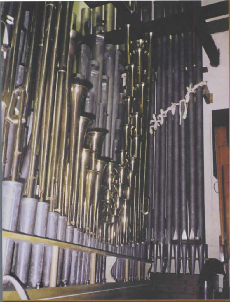
Above: Solo Chamber / Maloof Residence Below: The grandest of them all starts taking shape.
