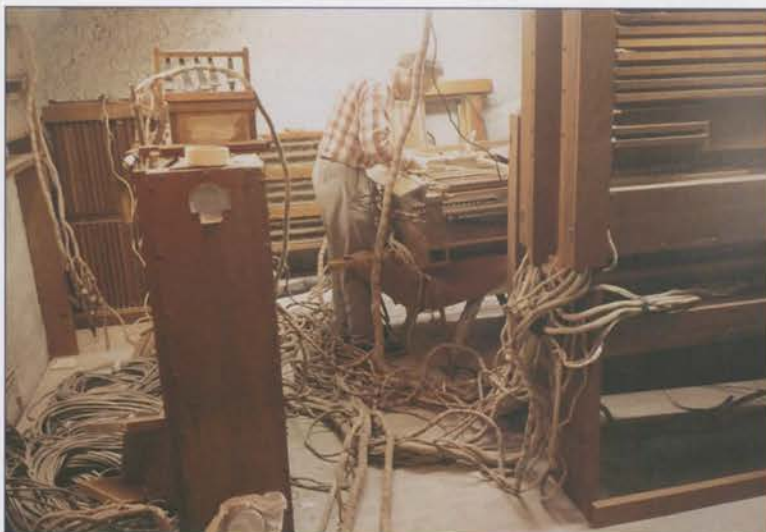
Sherrill Collins just starting to wire the Relays.
