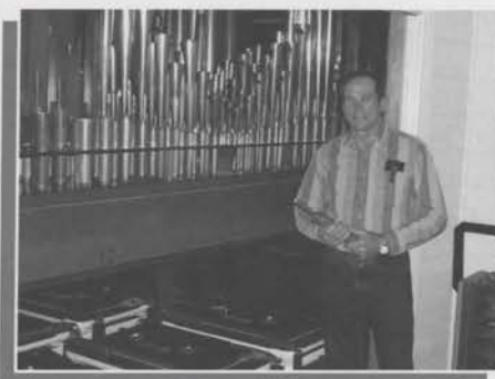
Chapter President Phil Lyons, Jr. standing beside the solo chamber of his expanded Wurlitzer 2/15 home installation.
