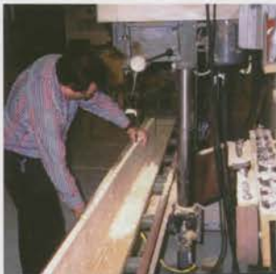
Boring holes in a new chestwork component.
