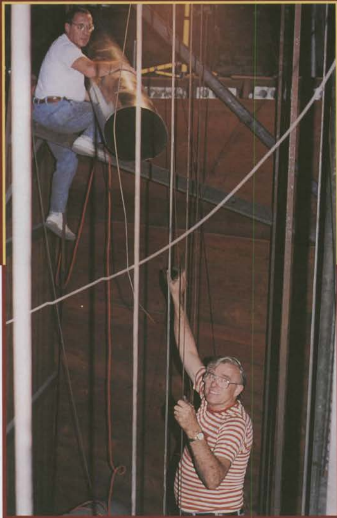
Ron Vaillancourt and Bob Martin hoisting in replacement windline over proscenium.
