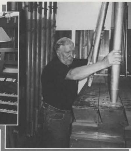
Restorer, Don Peterson, removes last two pipes from Main chamber chests to tackle needed repairs.
