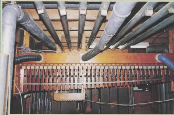
Xylophone and horizontal bass string pipes. Also, treble flute offset chest (below xylo).
