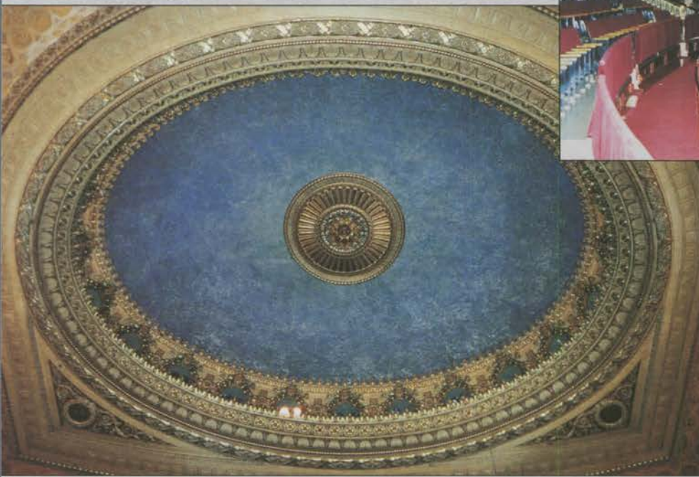
Large dome of auditorium ceiling. Note fine plasterwork around the circular openings.
