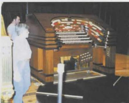
With the help of the orchestra elevator, the console is installed on the performance dolly.
