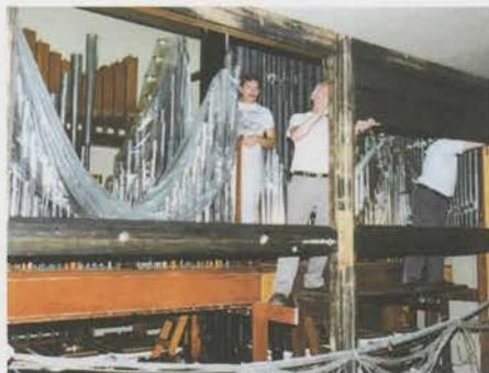
*The new solo shutter assembly was rigged piece by piece through the slots in the organ grille.*
