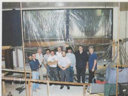
The solo chamber shutter wall has been removed and prepared for the new horizontal shutter assembly.
