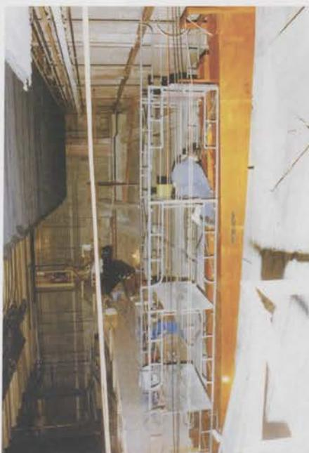
Two bold crew members avoid looking down as they work 60 feet above stage level to bolt the 32 foot wood diaphones to the back stage wall.
