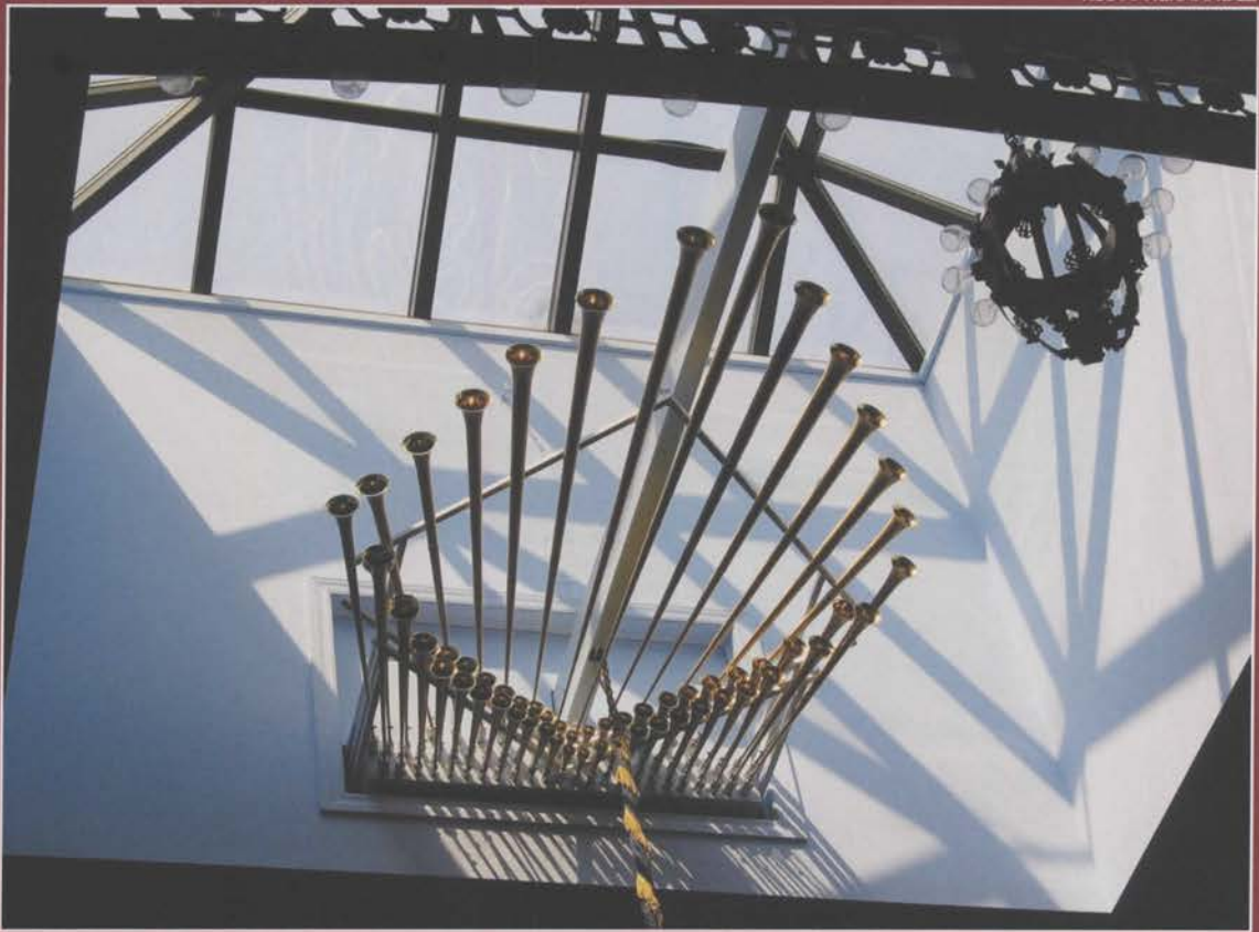
Trumpet Imperial rank mounted up in the light well of the main music room skylight.
