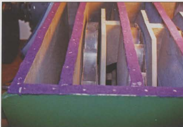
View of inboard bearing with cap off. This bearing has the new thrust bearing and spacer.
