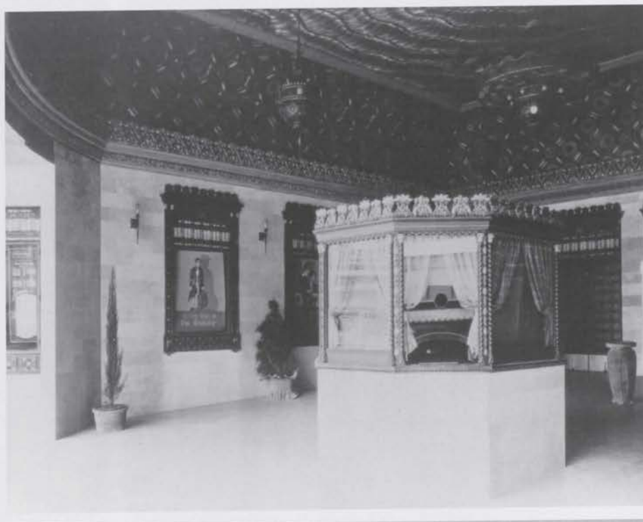
Right: The ceiling of the entrance was very elaborate, a typical Priteca touch. All San Diego photographs: Terry Helgesen Collection, THS.
