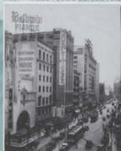
Looking south on Broadway in 1920s, one saw the Orpheum at end of "music row," with the Wurlitzer building prominent in middle of block.
