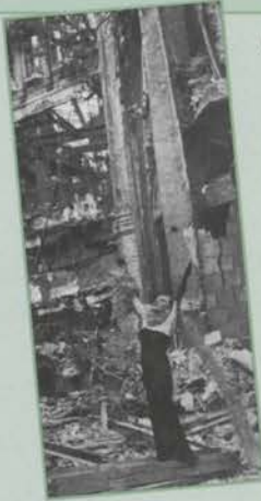
Heritage Lost: Gloria Swanson photographed at the (Paramount or Roxy) Theatre while under demolition.
