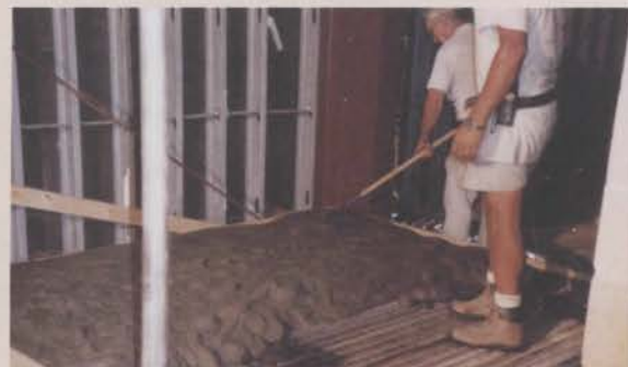
Pouring concrete for the newly created blower room.
