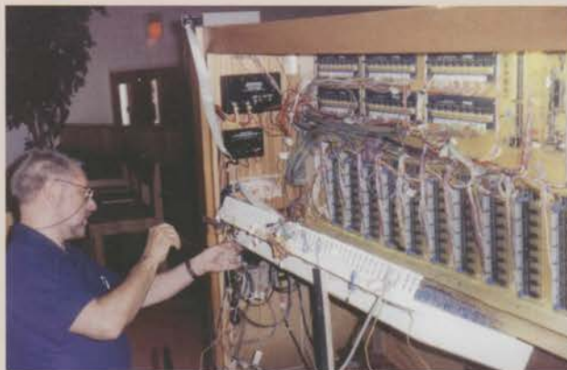
Allen Miller installing Z-tronics Relay System components into the new console.
