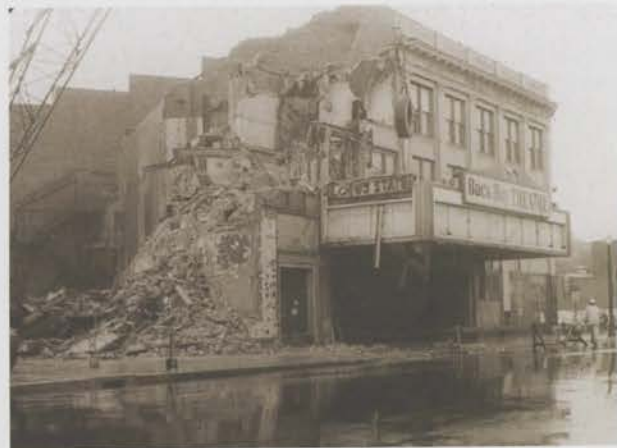
Partially Demolished Theatre.
